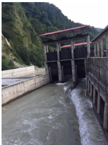
Intake of Lower Modi HEP
