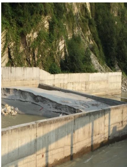
High rate of silt (east side of intake of Lower Modi HEP)
